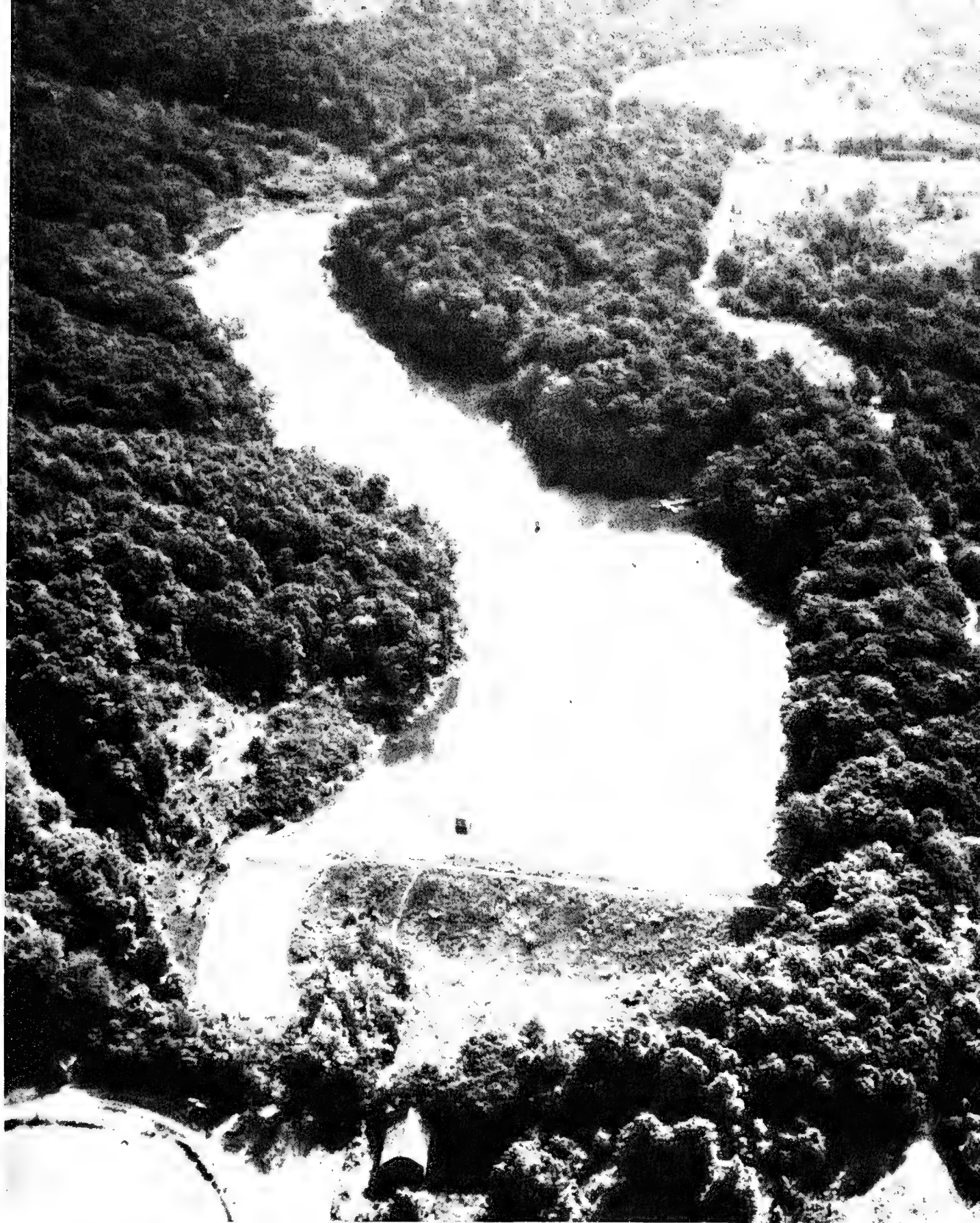
Aerial view of Ridge Lake, showing dam and spillway in foreground.
