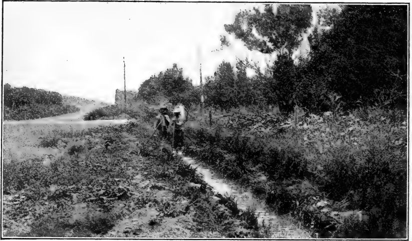
FIG. 9.—Cleaning a waste ditch in the Grand Valley district. This operation is necessary at least once a year and is one of the principal items of miscellaneous labor.
