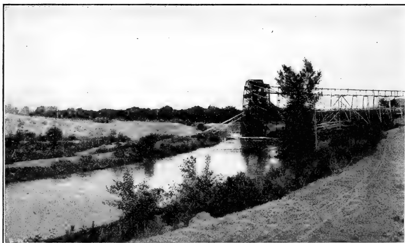
FIG. 8.—Method of raising water to irrigate lands above the Grand Valley canal near Grand Junction.
