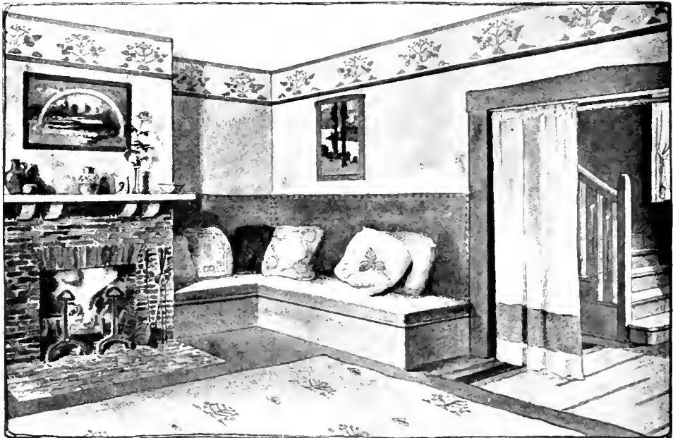
FIREPLACE AND SEAT IN THE LIVING ROOM, WITH GLIMPSE OF HALL AND STAIRCASE.
