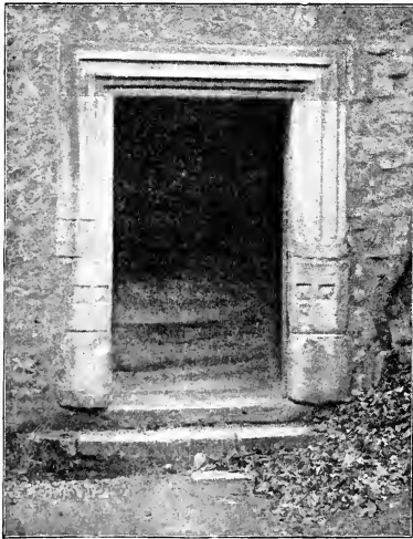
DOORWAY TO MAIN STAIRCASE.
