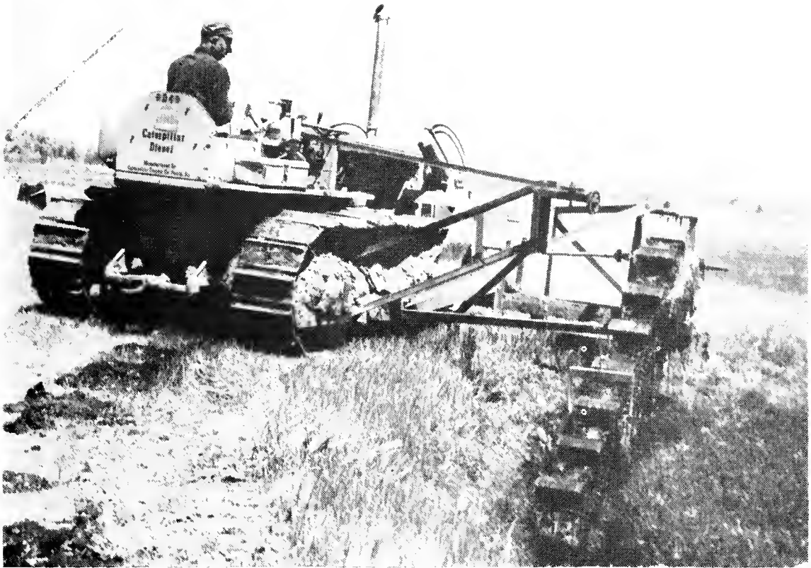
New Ditch Cleaner in Operation at Camp Douglas, Wisconsin. (CRANBERRIES Photo)
