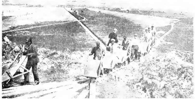
CONSTRUCTION WORK ON 235-ACRE BOG OF BURGESS CRANBERRY COMPANY
