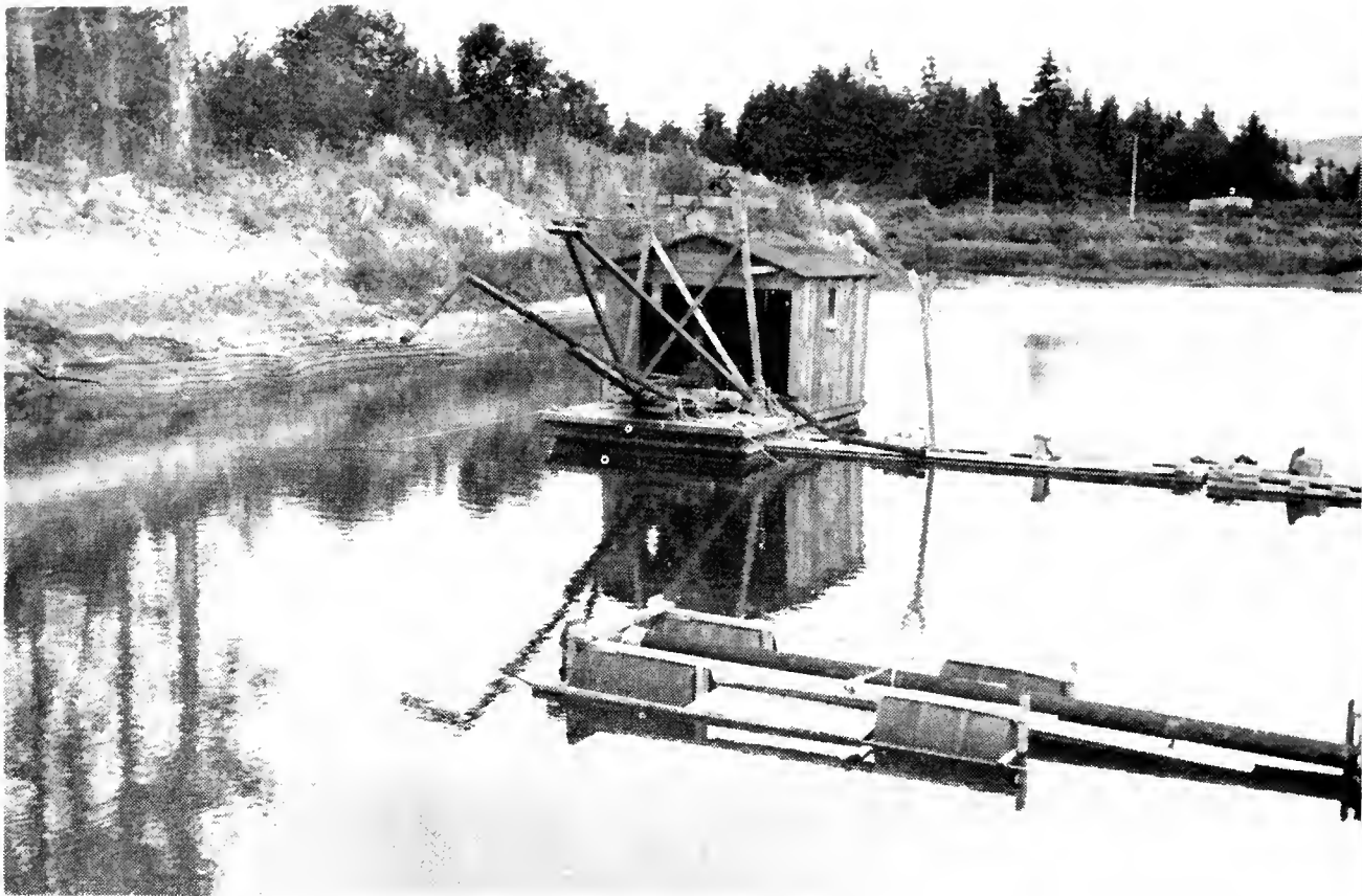
Above—View of the Morris bog sump and floating dumphouse
