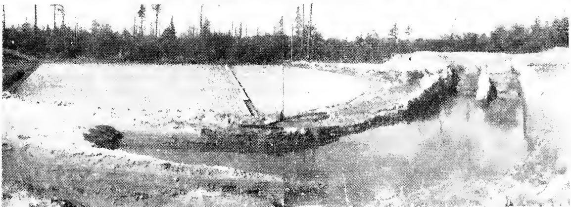
New bog in Oregon, center and marginal ditches are planked with part of center ditch covered with plank. Bundles of runners which were not used are still on the edge of the reservoir.
