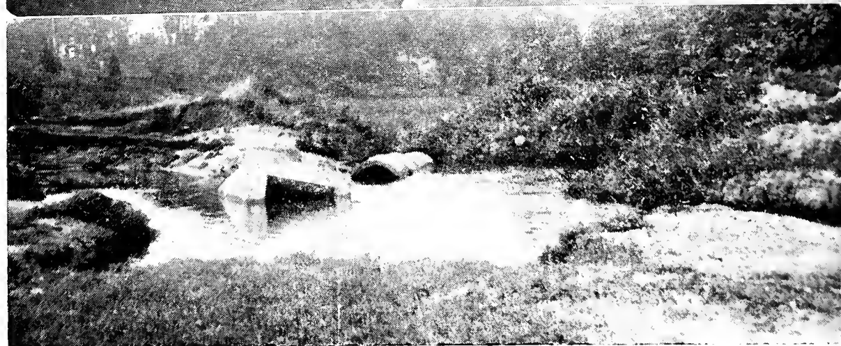
FIG. 2. The lower end of the Baker Bog, Buzzards Bay, showing the dike washed onto the bog. Nearly all of the fruit was washed from the vines. Figure 4 is the same bog from a different point of view. FIG. 3. Smith Hammond Company Bog in Onset. This dike washed away, part onto the bog.
