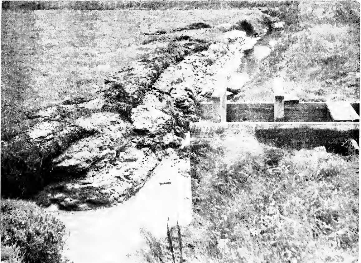
FIG. 1. The Smith Hammond Company Onset Bog. The water rushing over this dike washed under the cranberry sod and rolled it over. Also note erosion near flume. Figure 3 was taken from this dike. (All photos by Dr. Chandler)
