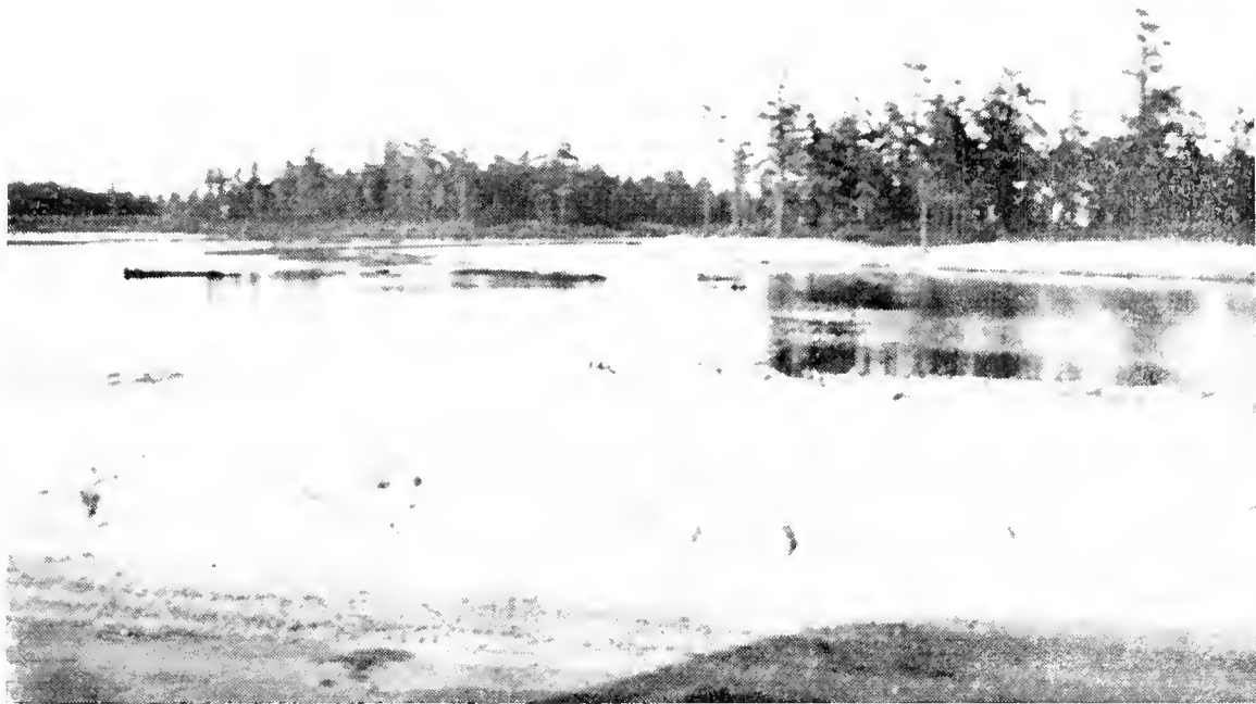
Method of converting reservoir, swamps and cranberry bog to a lake for housing and recreation.
