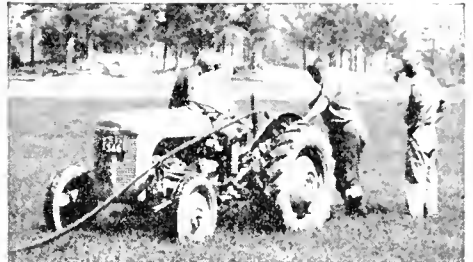
Carlon plastic drainage tubing can be installed at the rate of 4,000 feet in 50 minutes.
