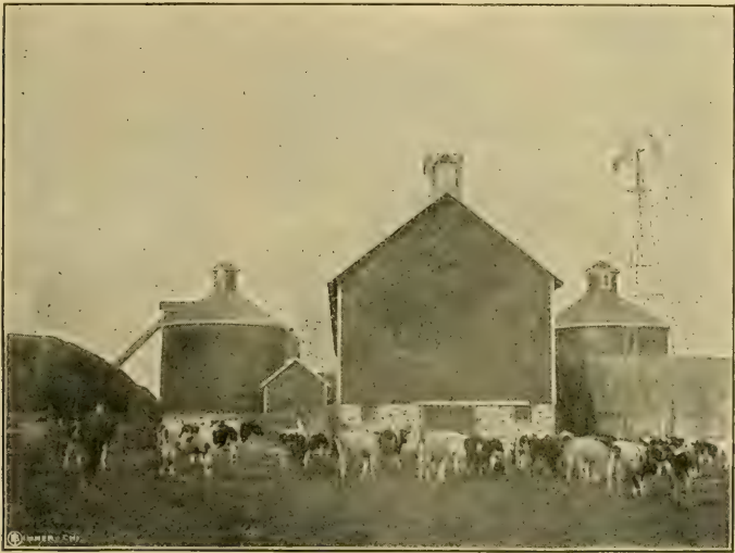
TWO ROUND SILOS WITH STONE FOUNDATIONS AT HUBBLETON, WIS.
