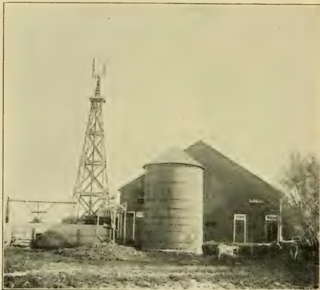
SILO WITH BOARD ROOF AND \frac{5}{8} INCH ROUND-IRON HOOPS.
