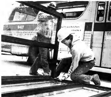
Attaching the back and side sections of the shelter.
