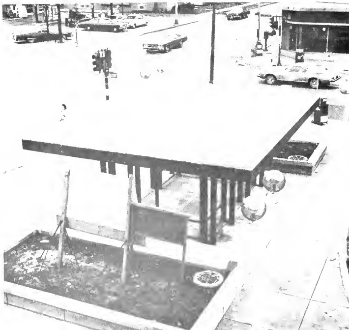
A NEW TURNAROUND: This $147,000 bus turnaround at Division and Austin is 90 per cent complete. Already in use, it still needs minor electrical work, painting and landscaping before work at the site can be finished. The turnaround provides facilities for employees as well as windscreens, lights and a pay phone for public use.
