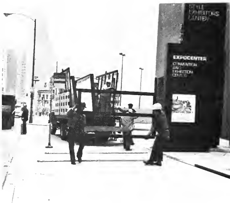
Unloading the prefabricated section of the bus passenger shelter.
