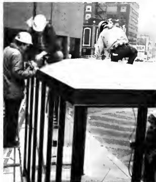
Attaching the roof to the sides of the shelter.
