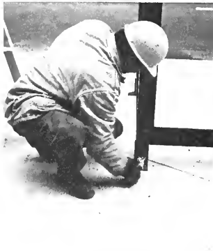
Bolting the shelter to the sidewalk.
