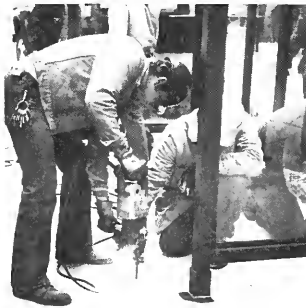
Drilling holes into concrete for bolting shelter to sidewalk.
