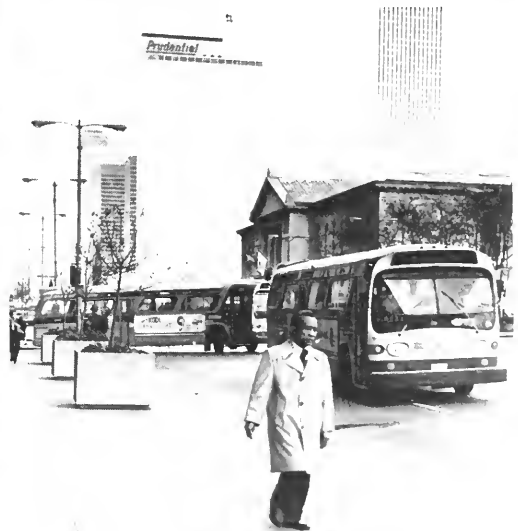
50-seat air conditioned diesel buses (1972 to present)
