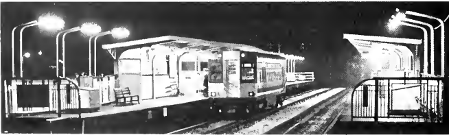
New lighting at Davis station on the Evanston 'L'
