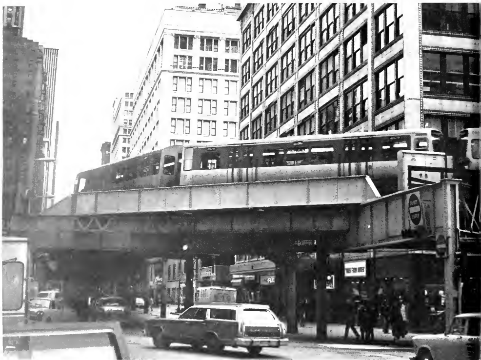
The 12-ton barrier on the Wabash and Lake curve of the Loop 'L' was built and installed in one weekend. It is shown above, painted, and in Monday morning service. (Photo by Bert Calvey)
