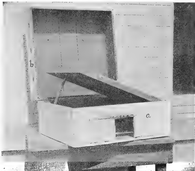
FIG. 171.—A cheap but efficient fireless brooder: a , Box; b , hinged lid showing ventilator openings; c , the removable frame, covered with cheese-cloth and on which a sack of feathers or woolen blanket may be placed as an overhead protection. This cheese-cloth is made to sag in the center.
