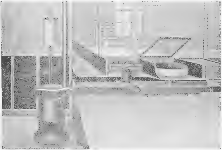
FIG. 177.—A view of the heating system of the giant brooder system, showing hot-water pipes, heat drum, and hover.
