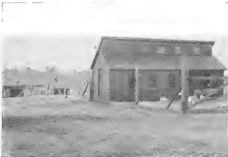
FIG. 66.—A partial view of a poultry plant, showing at a a half monitor house; b , two-thirds span house; c , a shed roof house; d , an outdoor dry mash hopper.
