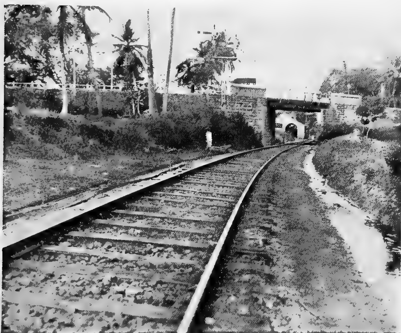
Fig. 42. Breeding places of Anophelines. Railway cutting at Kurunegala. The water course flowing on each side of the permanent way supplying the engines with water. These channels are blocked with weeds, from amongst which larvæ of A. culicifacies and A. rossii have been taken. After Bahr (from the Tropical Diseases Bulletin ).
