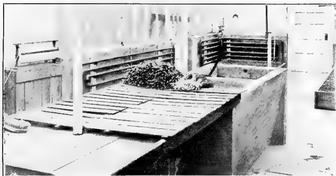
Fig. 58.—Corner of packing room in a well-managed establishment.
