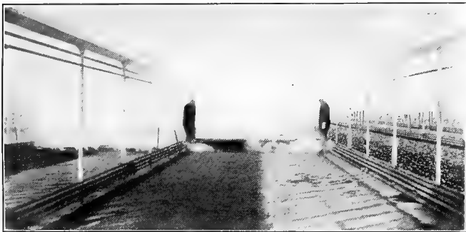
Fig. 32.—Peg steam sterilizer in operation at Toledo, Ohio.
