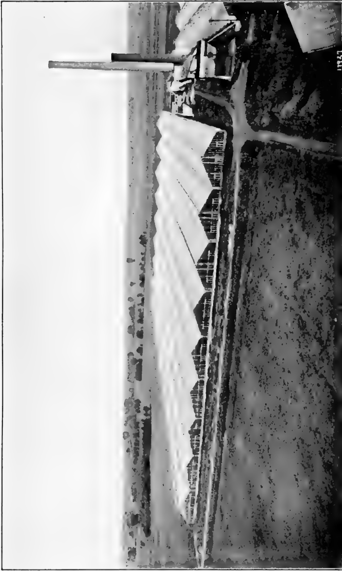
FIG. 7.—EVEN-SPAN HOUSES WITH CONTINUOUS VENTILATORS
