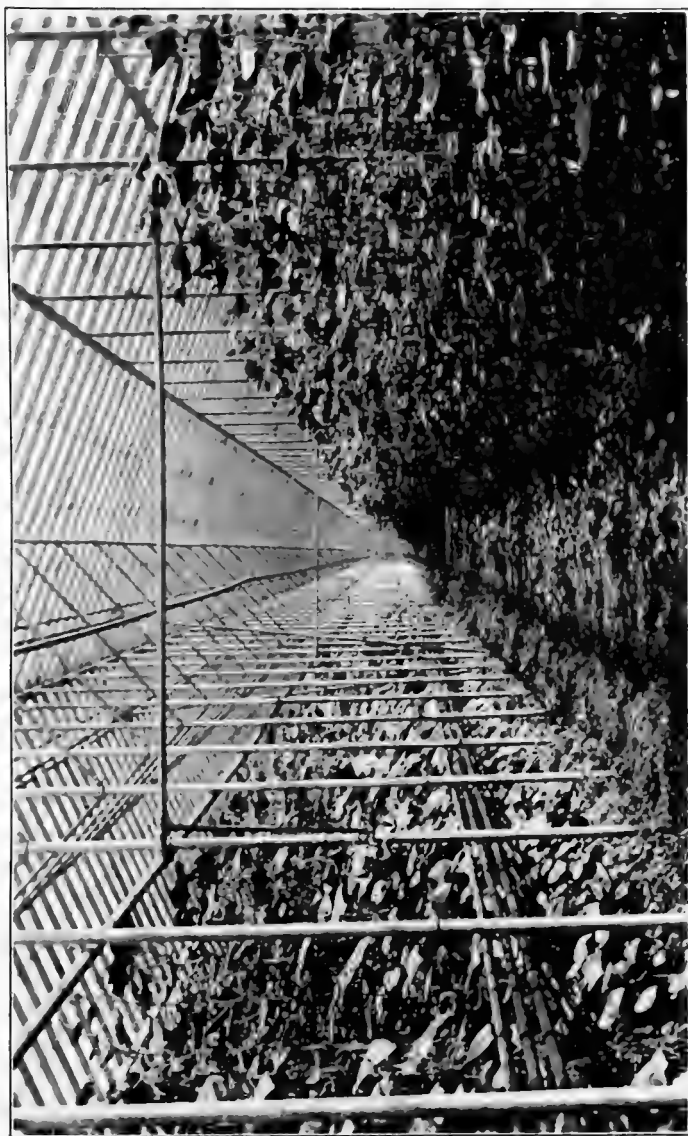
FIG. 25.—ROADWAY IN A TWO-ACRE HOUSE.
