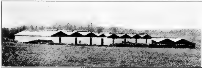
Fig. 148.—A modern commercial mushroom range at Kennett Square, Pa. Built of concrete and tile. Frostproof and fireproof.
