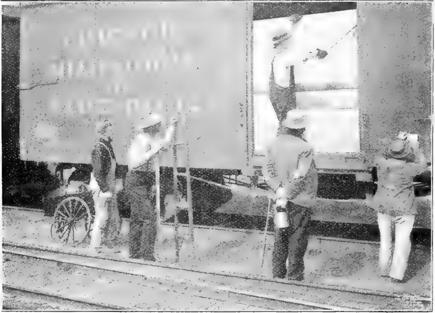
THE EXTRA BOARDS ARE BEING REMOVED
