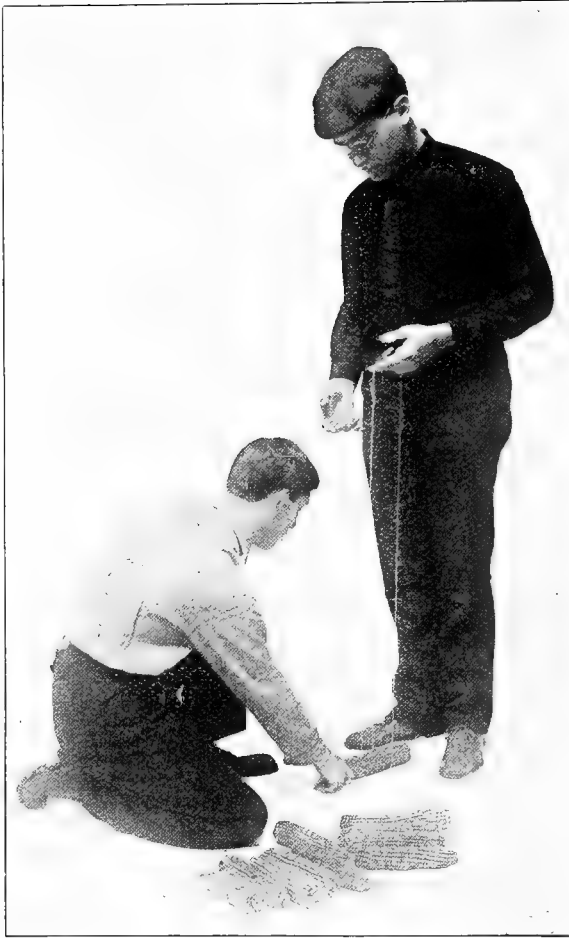
LAYING IN THE FIRST EAR
