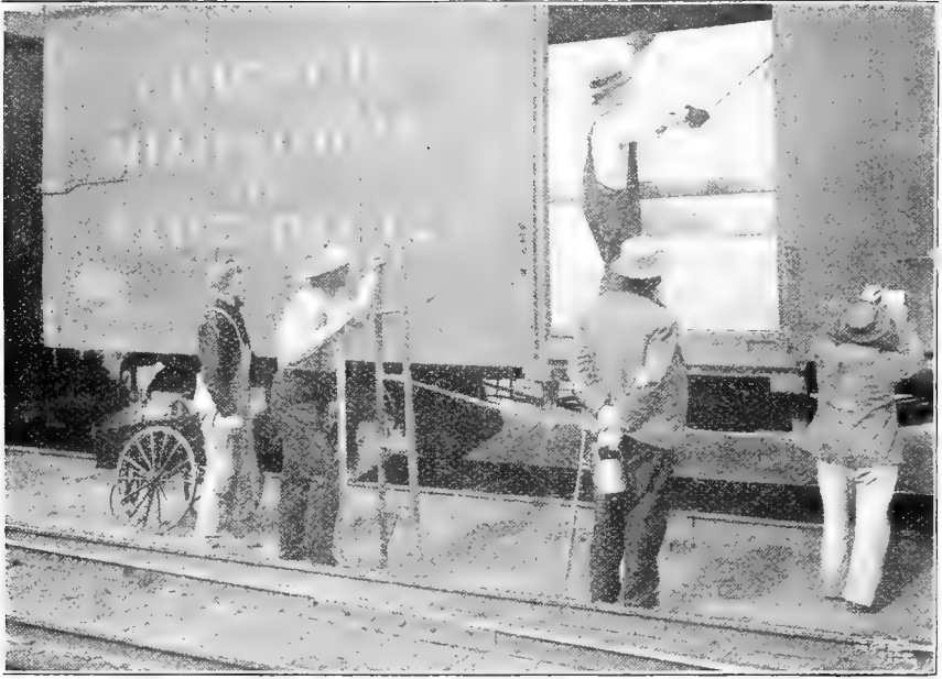
THE EXTRA BOARDS ARE BEING REMOVED
