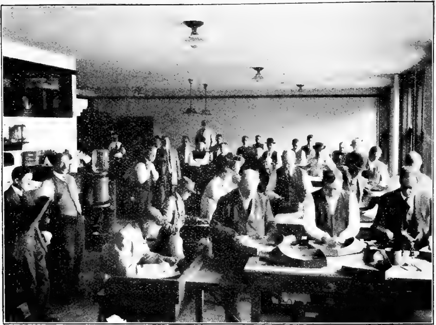
THE MAIN INSPECTION ROOM. (Illinois Inspection Department)
