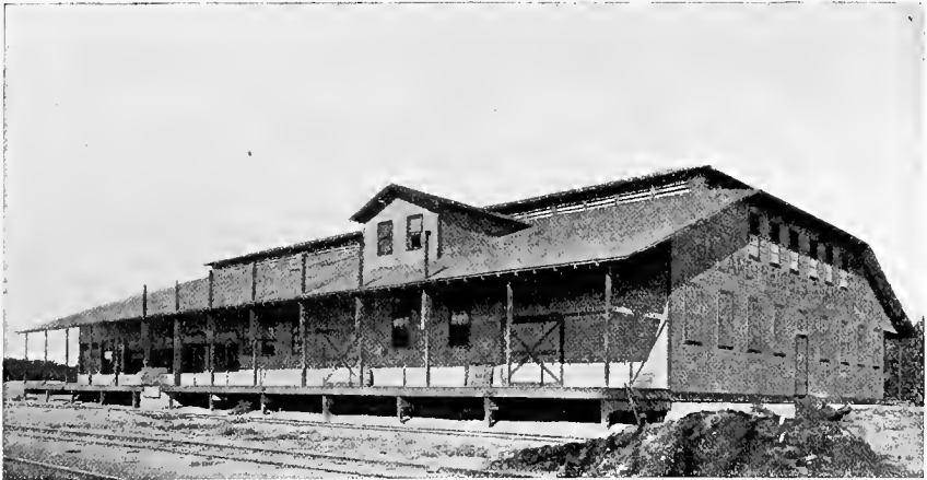
FIG. 1—FRUIT PACKING HOUSE AND PRE-COOLING PLANT, UPLAND HEIGHTS ORANGE ASSO., UPLAND, CAL.
