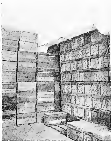
FIG. 2.—EGG ROOM—FALSE FLOOR AND FALSE CEILING SYSTEM OF COOLING.
