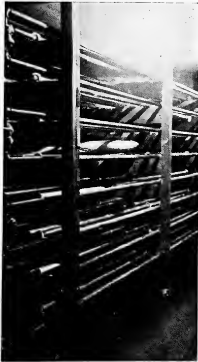
FIG. 2—SHARP FREEZER FOR FISH.—PIPES HAVE BEEN CLEANED PREPARATORY TO RECEIVING A NEW BATCH OF FISH IN PANS.
