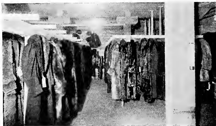
FIG. 7.—FUR STORAGE ROOM—COOLED BY FAN SYSTEM OF AIR CIRCULATION—NO PIPES IN ROOM.—FRANKLIN REFRIGERATING COMPANY, SARANAC LAKE, N. Y.
