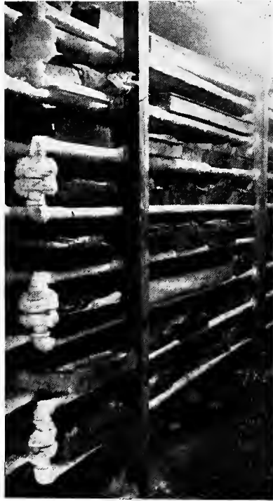
FIG. 3—SHARP FREEZER FOR FISH.—THE PANS IN THIS CASE CONTAIN STURGEON TO BE FROZEN.
