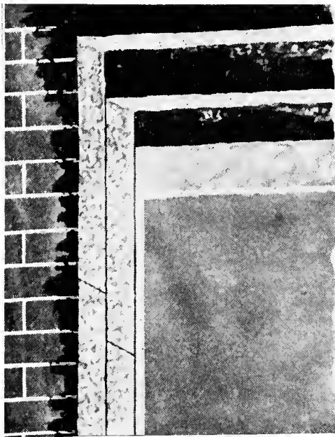
FIG. 11—METHOD FOR APPLYING MINERAL WOOL SLABS.
