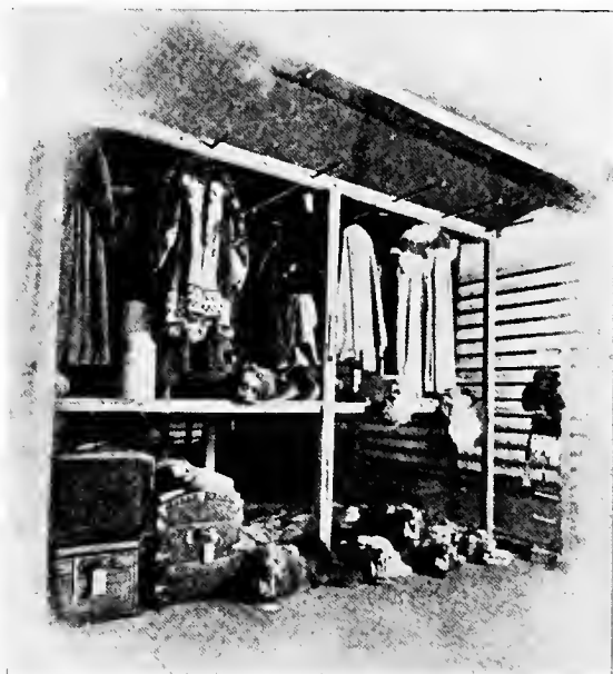
FIG. 2.—COLD STORAGE ROOM FOR FABRICS AND TROPHIES, SHOWING COOLING PIPES.
