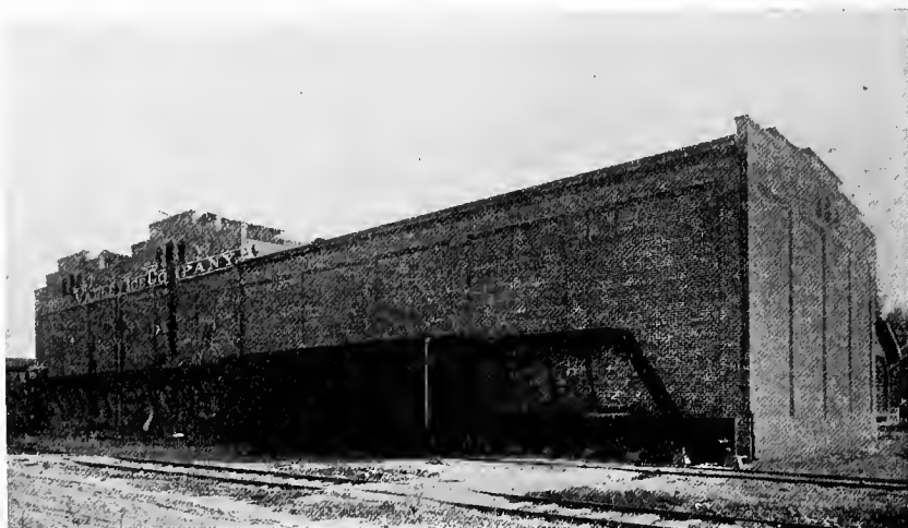
FIG. 8—POMONA VALLEY ICE CO. PRE-COOLING PLANT. Railroad side showing platform on which ice is brought from ice storage to the left and loaded into the bunkers of refrigerator cars.
