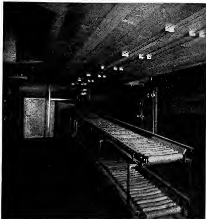
FIG. 15—VIEW IN CORRIDOR IN BASEMENT.
