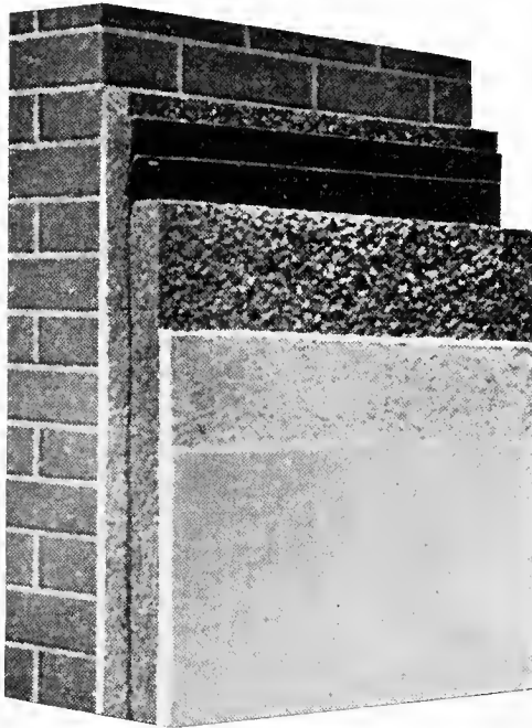
FIG. 12—SHEET CORK INSULATION WITH CEMENT PLASTER FINISH.
