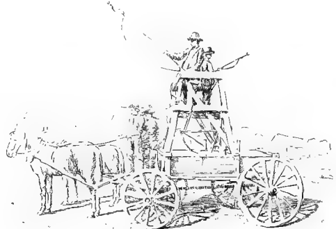
2378. Orchard pump with conical tower rig.
