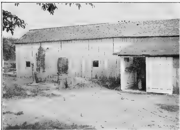
MILK HOUSE CONNECTED WITH THE STABLE—A BAD PRACTICE
