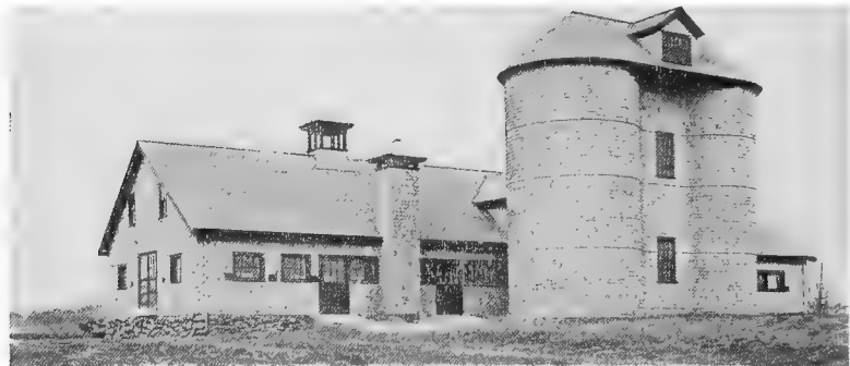
FIG. 75.—Art and utility may be successfully combined. Dairy stable and two silos belonging to E. H. Sears.
