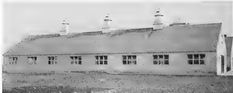
FIG. 85.—A well-lighted dairy barn. Note that top sash of windows fall inward to aid in ventilation. Owned by H. P. Hood and Sons, Boston. (Courtesy of James Mig. Co.)
