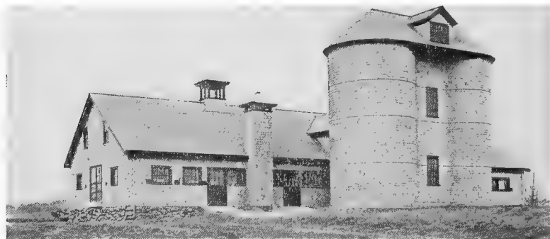
FIG. 75.—Art and utility may be successfully combined. Dairy stable and two silos belonging to E. H. Sears.
