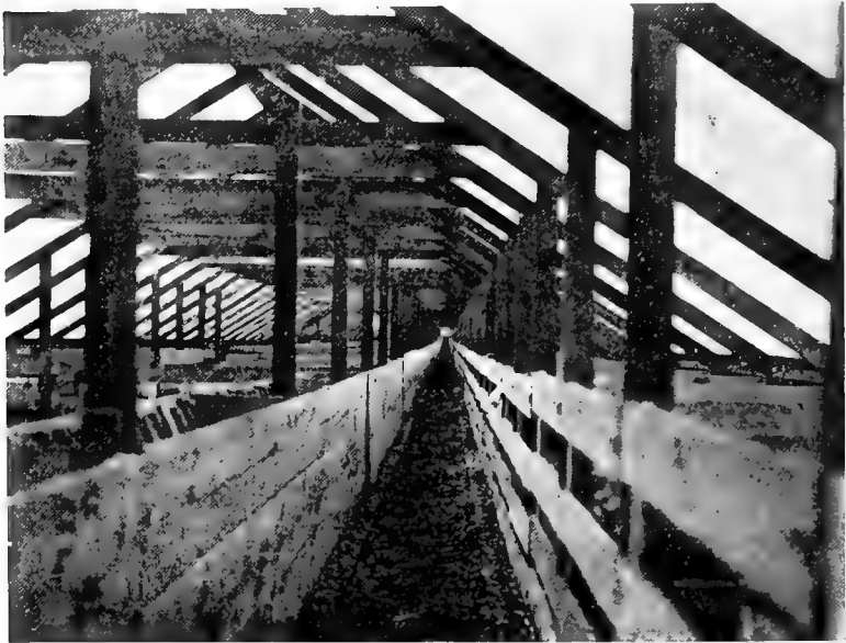
FIG. 231.—A permanent lambing camp consisting of a wooden frame and canvas roof and walls.
