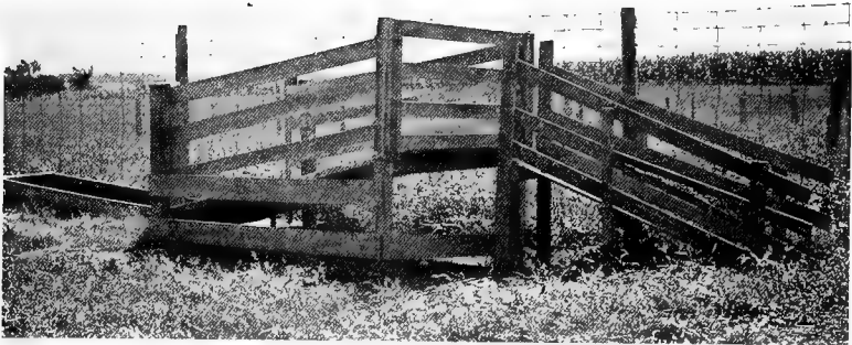
Fig. 249.—Farm dipping plant. Tank to the left; dripping pen in center, and chute from dripping pen at the right.
