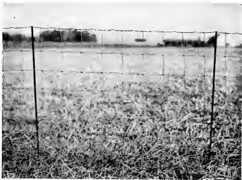
FIG. 251.—Temporary fence supported by iron posts.
