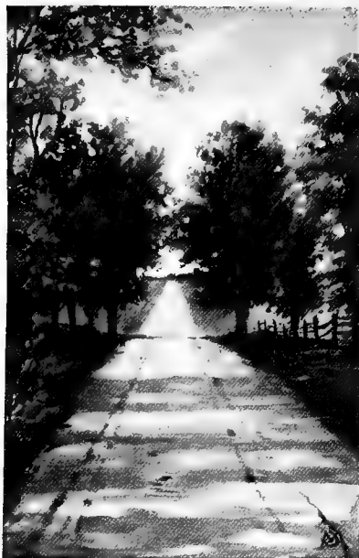
ROAD NEAR DODSONVILLE, HIGHLAND CO., OHIO.
