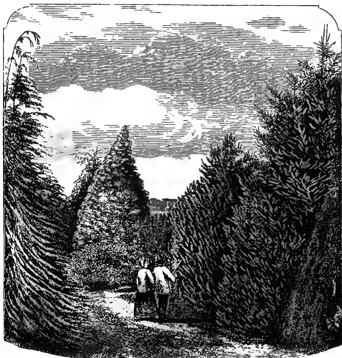
EVERGREEN-WALK IN PARSONS' NURSERY, FLUSHING, L. I.
