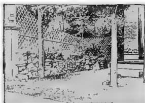
A lattice screen, supported at the base by a wall. Between the chinks of the stones and in a channel along the top, suitable plants are grown
