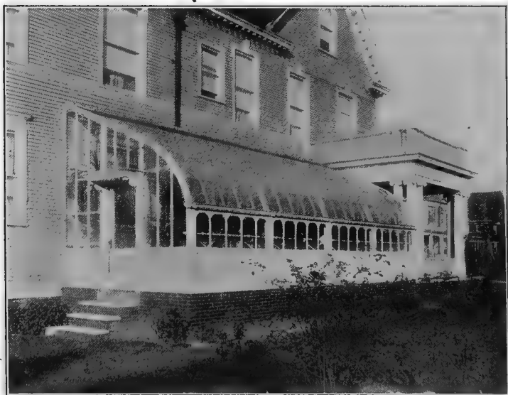
A curvilinear roofed, lean-to conservatory by Hitchings & Co., with substantial brick foundation
