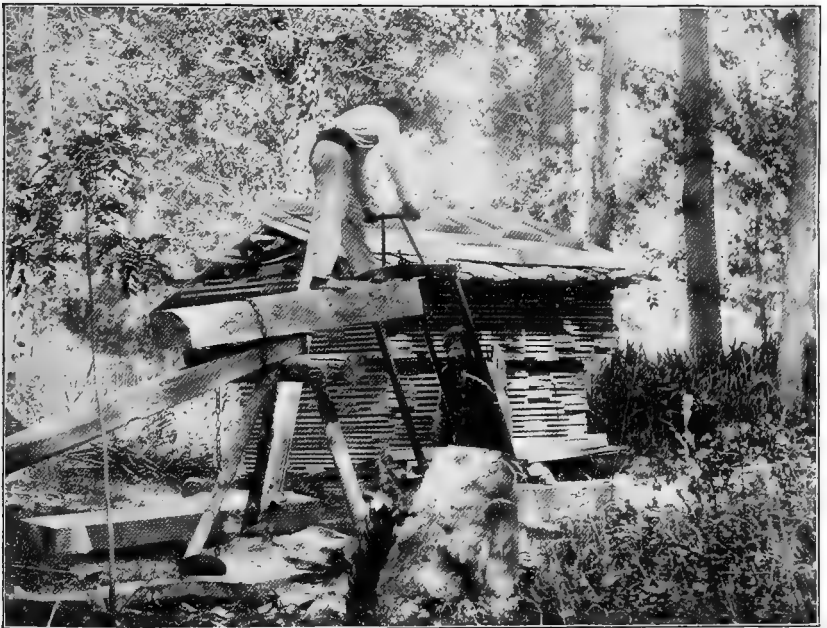
SAWING BOARDS BY HAND IN FRANCE
