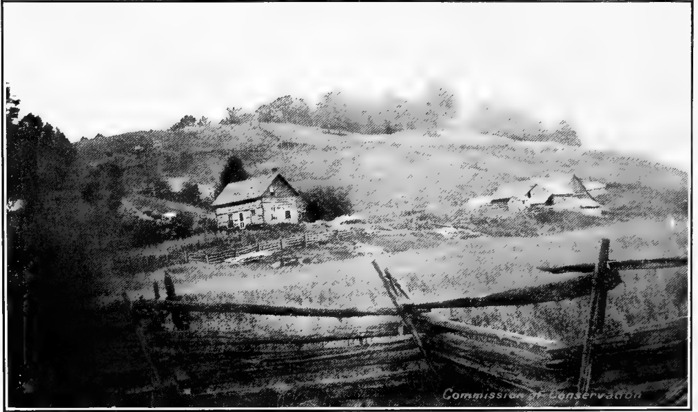
TYPICAL UPLAND FARM AND FARM BUILDINGS
