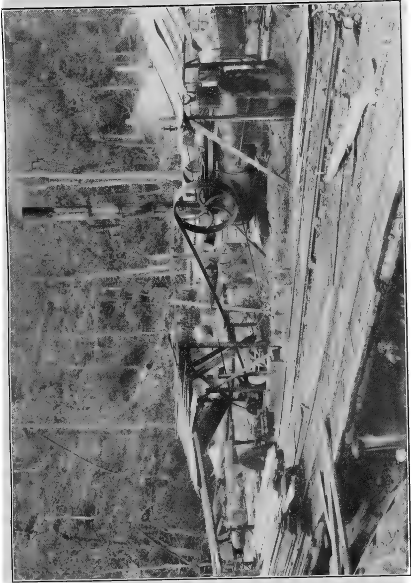
Portable sawmills cutting 5,000 or 10,000 board feet a day, do not as a rule manufacture lumber of as good a quality as they should. The quality could usually be much improved by efficient handling, careful sawing, and attention to the grade.
