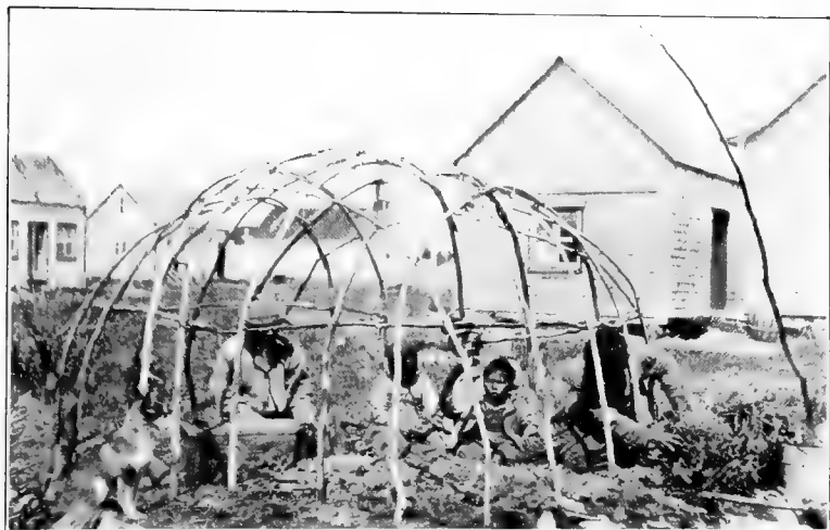
WIGWAM IN PROCESS OF CONSTRUCTION AT MINGAN.
