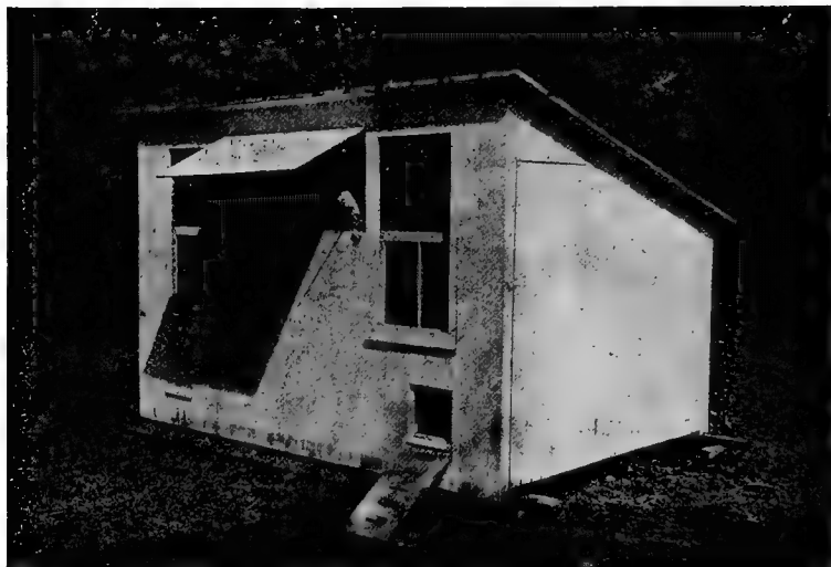
Fig. 218.—Inexpensive colony growing coop built on skids.
