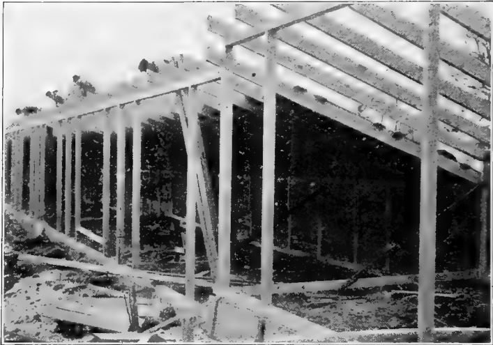
Fig. 86.—Framing for a continuous poultry house. Note the concrete walls; building is intended to have a dirt floor.
