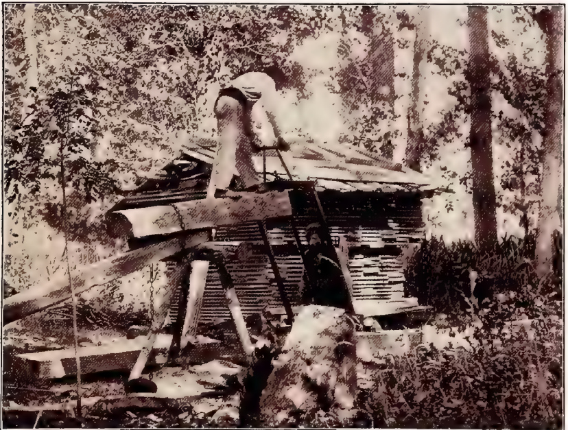
SAWING BOARDS BY HAND IN FRANCE
