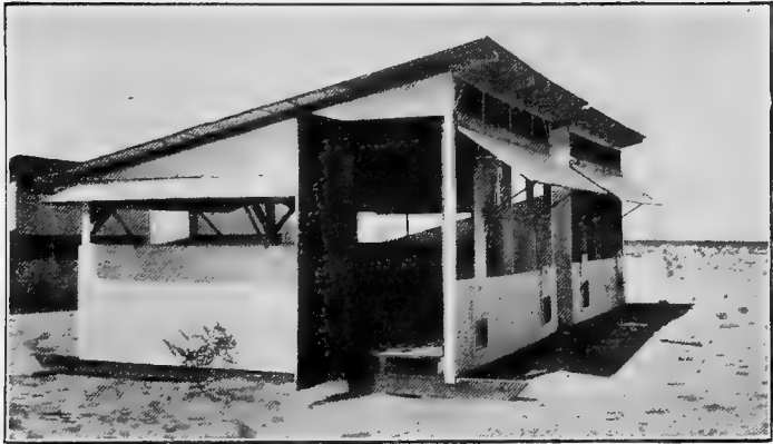
Figure 128.—Type of house suitable for a hot climate. Note the openings in the front, sides, and back to provide ample ventilation.
