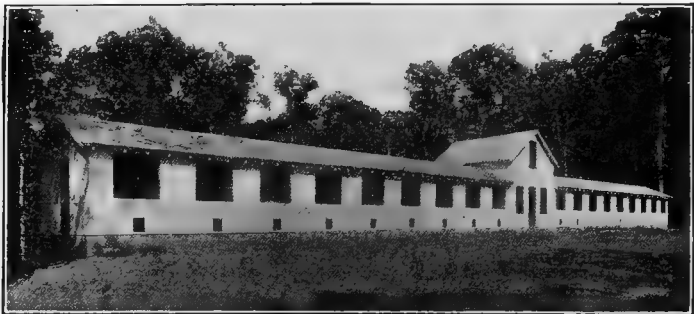
Figure 146.—The continuous house completed.
