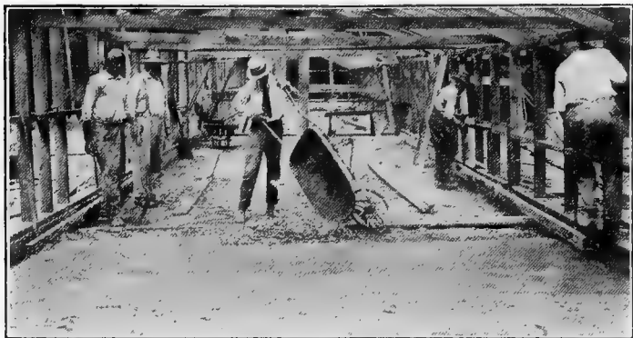
Figure 130.—Laying a concrete floor in a continuous house.
