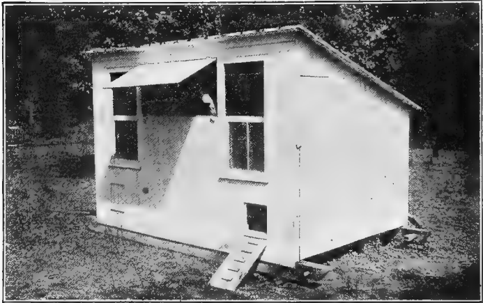
Figure 122.—A practical easily constructed colony house that will accommodate a flock of 25 fowls.
