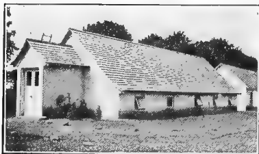
Figure 79.—An exterior view of an incubator cellar on a commercial poultry farm.
