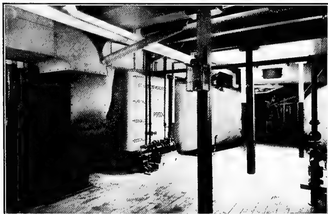
FIG. 108.—Tanks for bichloride of mercury, government quarantine disinfecting plant.
