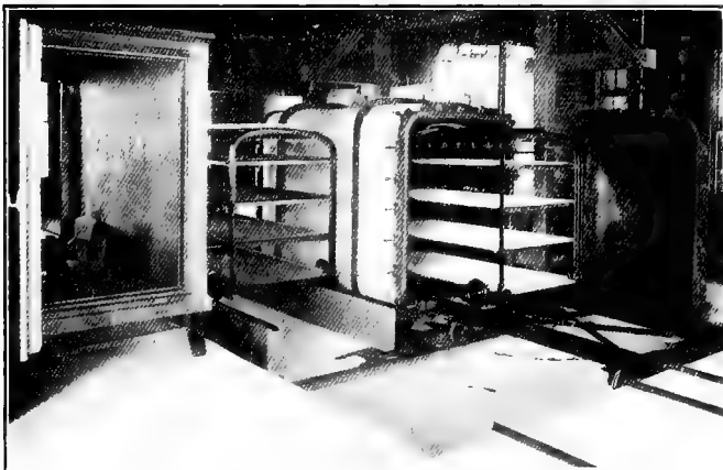
FIG. 90.—Municipal disinfecting station, Washington, D. C.
