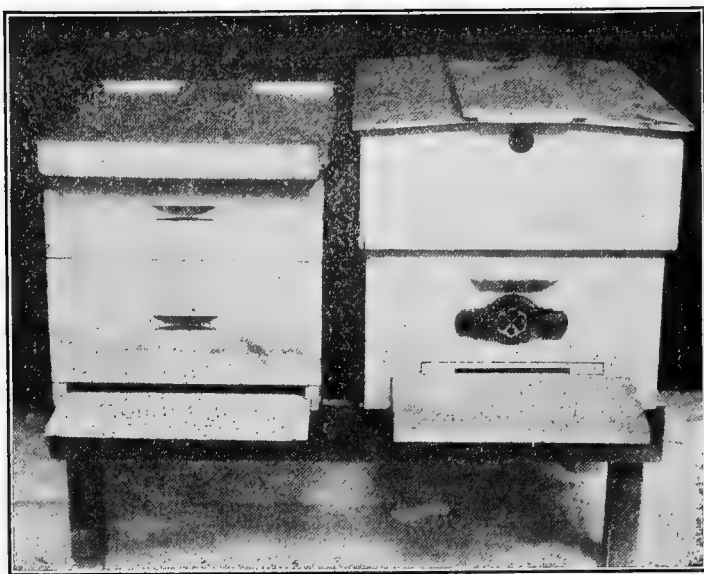
FIG. 16—A SINGLE AND DOUBLE-WALLED HIVE
