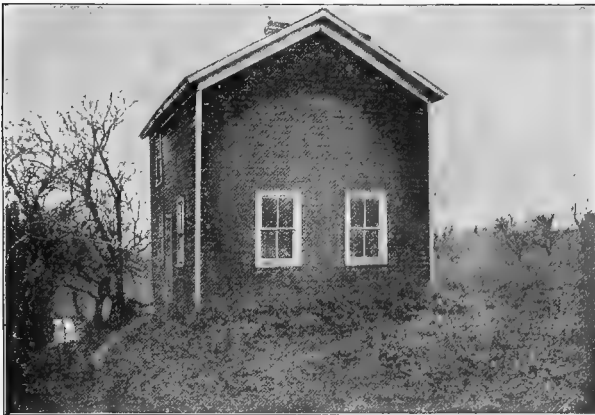
Fig. 71.—Shop (looking South).
