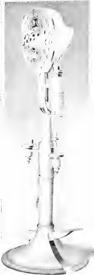
FIG. 25. The foot milk bottle crowning machine.
