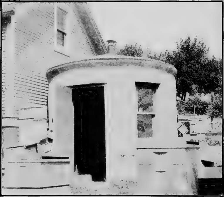
Fig. 27. A cylindrical honey-house made especially for storing combs by hanging them in racks so the moths will not enter them, and also for using sulphur fumes. Apiary of H. C. Cook of Omaha.
