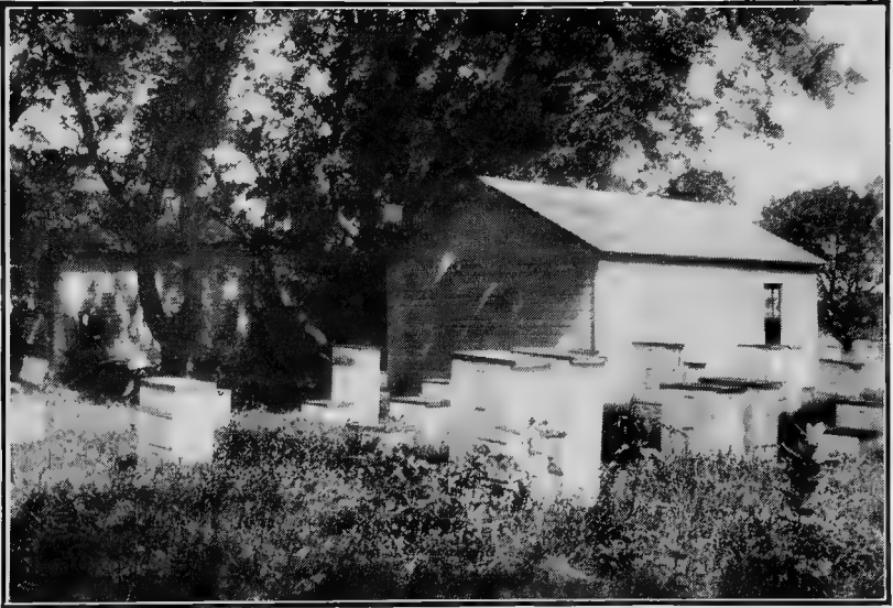
Fig. 54. Honey-house built so that it may be readily cut apart into sections and removed. Where the cut is to be made, rafters or studding are placed within an inch of each other and holes bored so that the sections may be drawn together with bolts when set up again.
