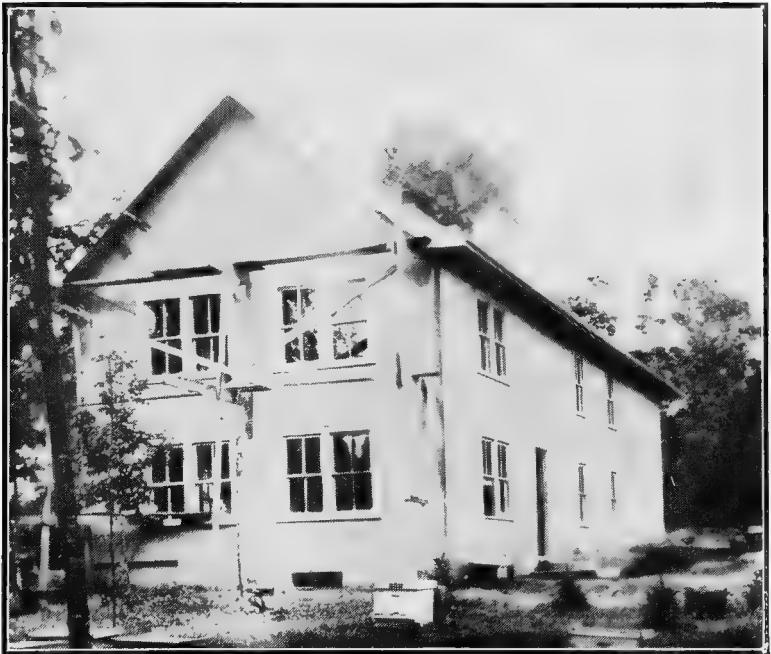
Fig. 58. Central plant of the Jager apiaries in Minnesota. This is one of the most complete buildings of its kind anywhere.
