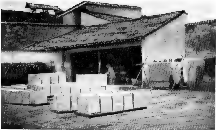
LEAD LININGS FACTORY
