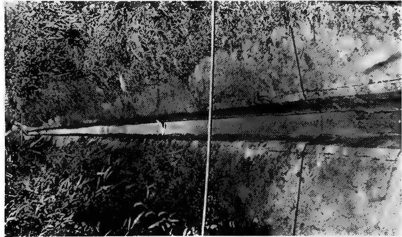
Concrete lining of a ditch of small cross-section
