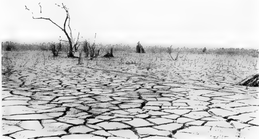
Cracks in a hydraulic fill
