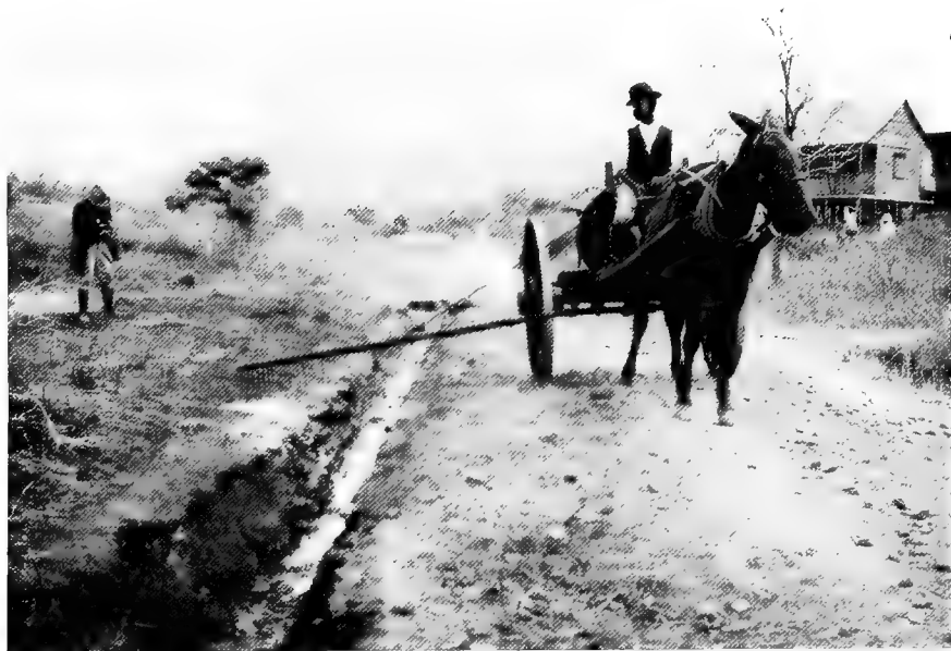
Oil cart for applying oil to roadside ditches
