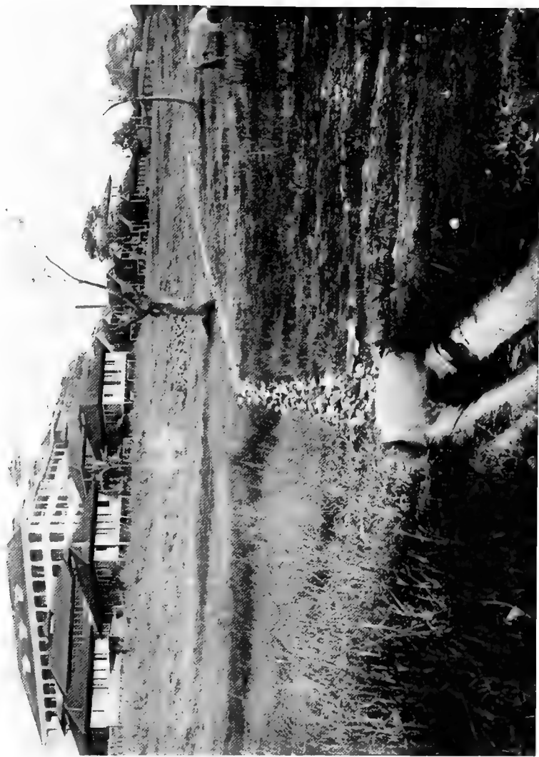
A seepage outcrop, controlled by an intercepting tile ditch: Ancon
