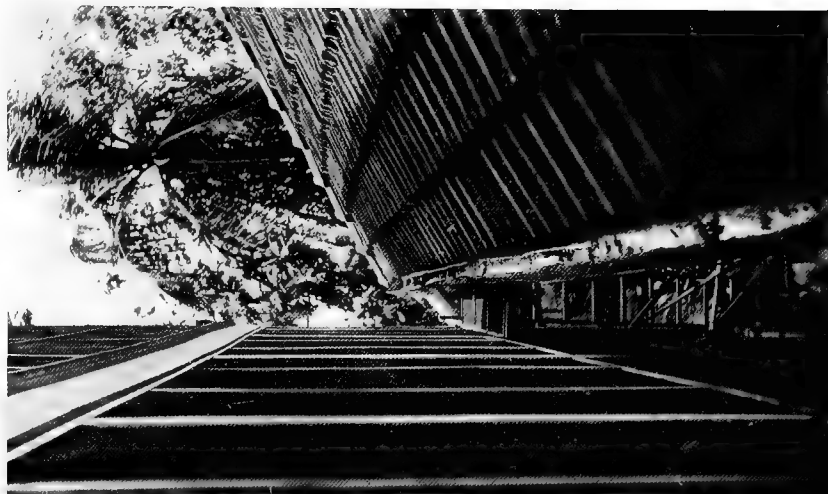
A poorly constructed eave trough
