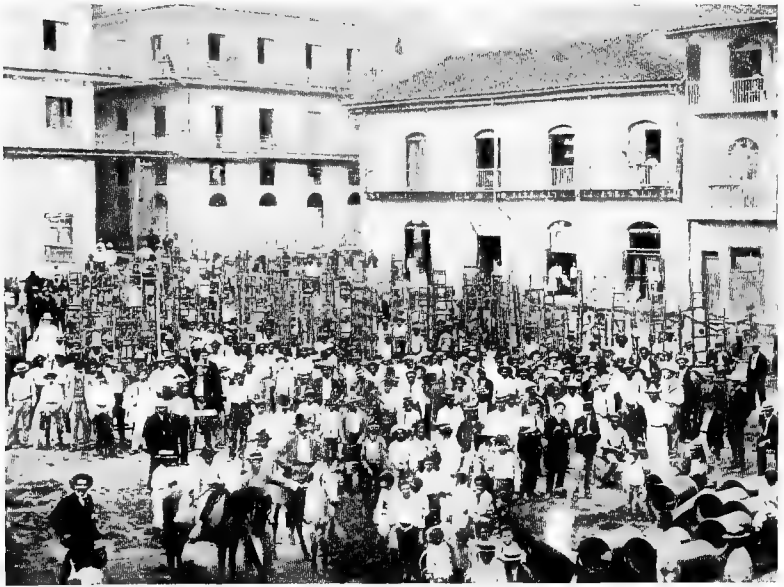
Part of the Panama fumigation brigade
