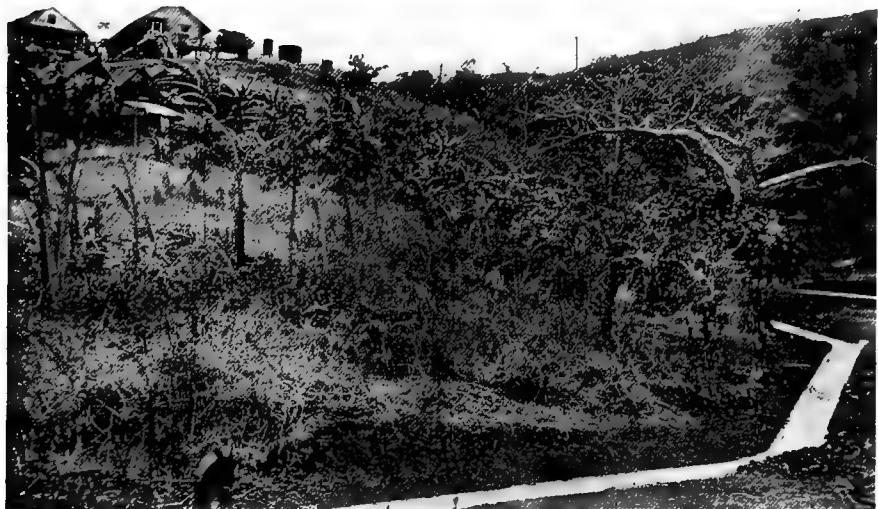
Concrete-lined ditch at Balboa
