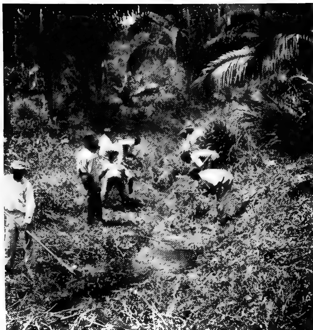
Removing vegetation from overgrown streams: Machetes are used
