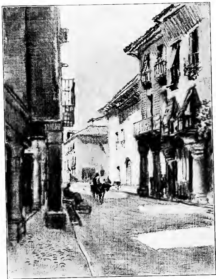
CALLE MAJOR, ALCALÁ
