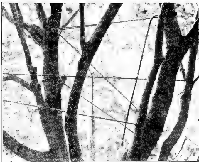
FIG. 311 ROPING A TREE PREPARATORY TO BOLTING
