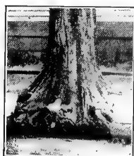
FIG. 302—MUTILATED TO LAY A CURB
