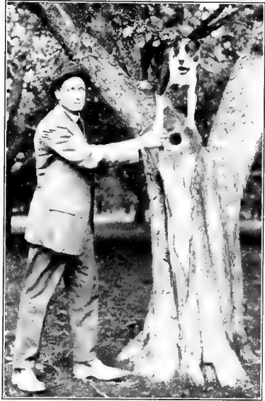
FIG. 2—WRONGLY CUT LIMB WITH DECAY HOLE
