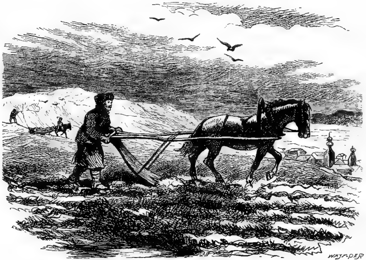
PLOUGHING AT UST-ZYLMA
