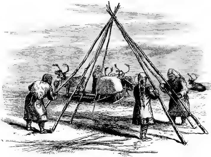
SAMOYEDES ERECTING A CHOOM
