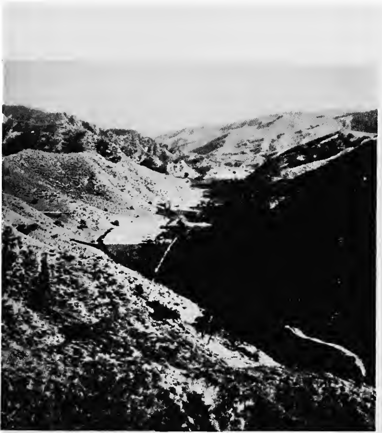
View south from over the San Fernando tunnel—Southern Pacific Railroad
