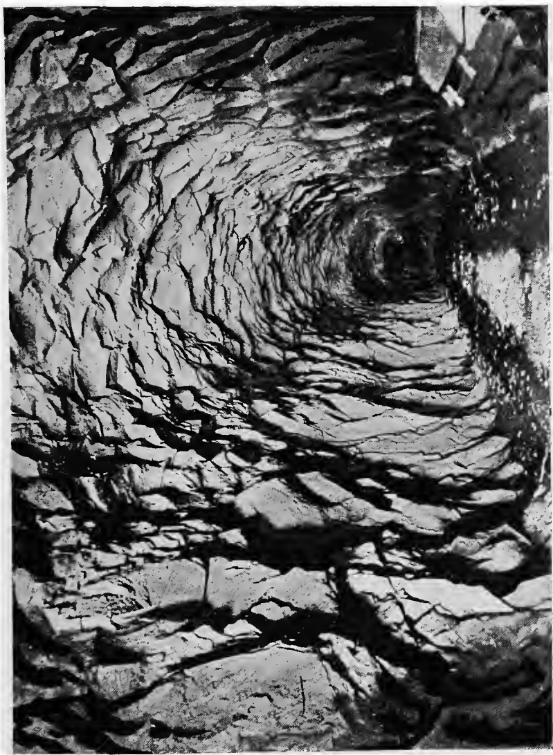
Summit tunnel (altitude 7,042 feet) before completion—Sierra Nevada Mountains
