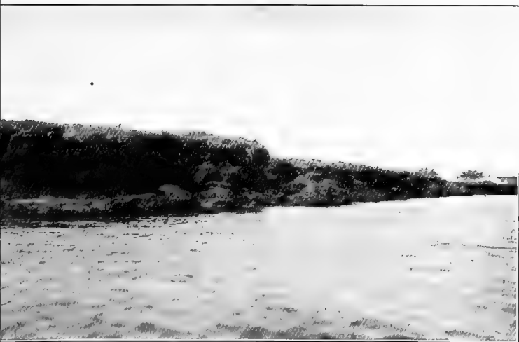
THE BANK FALLING AWAY ON THE CHANNEL SIDE OF A CREEK.
