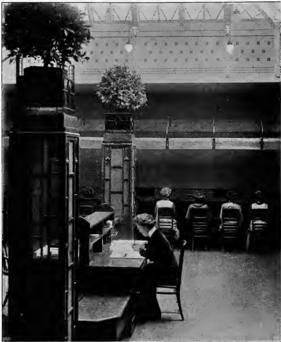
Local Station (Östermalm) of the Stockholm Telephone Co.
