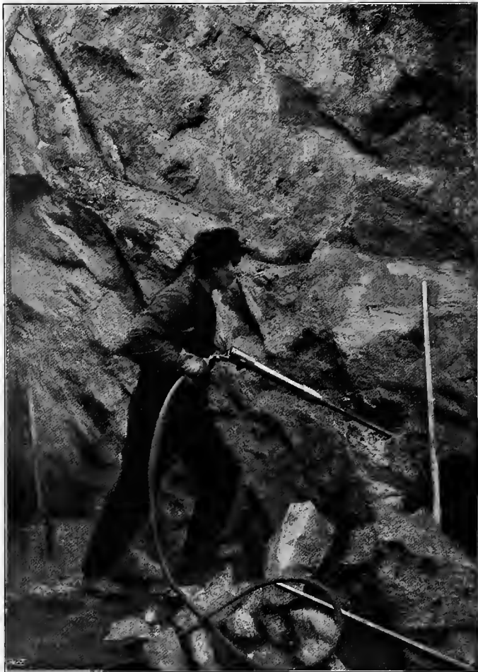
Swedish Hammer-drill Machine.
