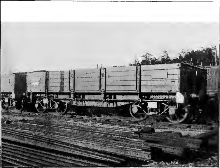
Open Freight-goods Bogie-car, State-Railways.
