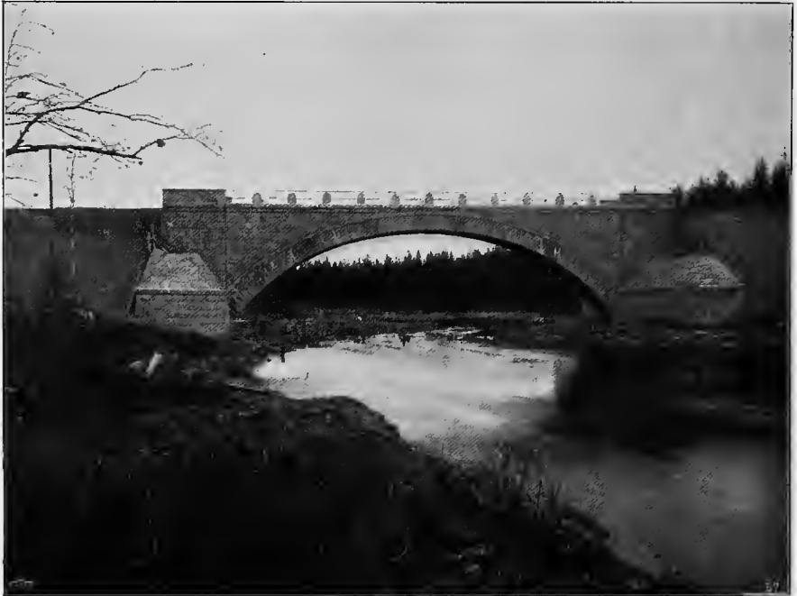
Railway-bridge (of granite) over the Flåsjöälven.
