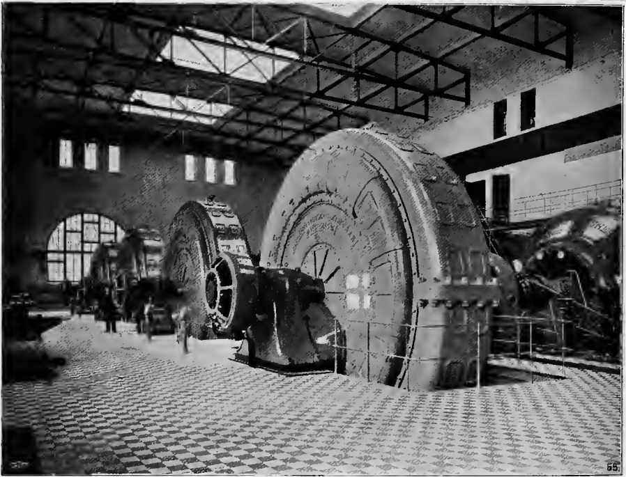
The Generator House of the Trollhättan Water-Power Station.
