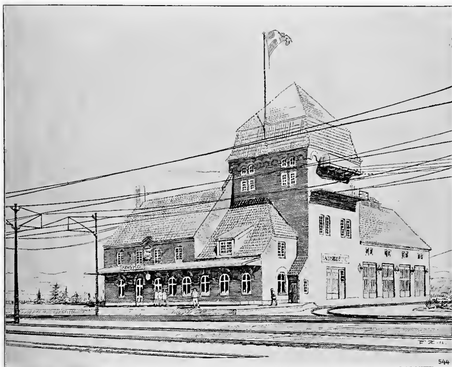
The Railway- and Transformer-station at Abisko (Kiruna—Riksgränsen).
