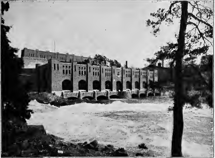
The Trollhättan Power Station.
