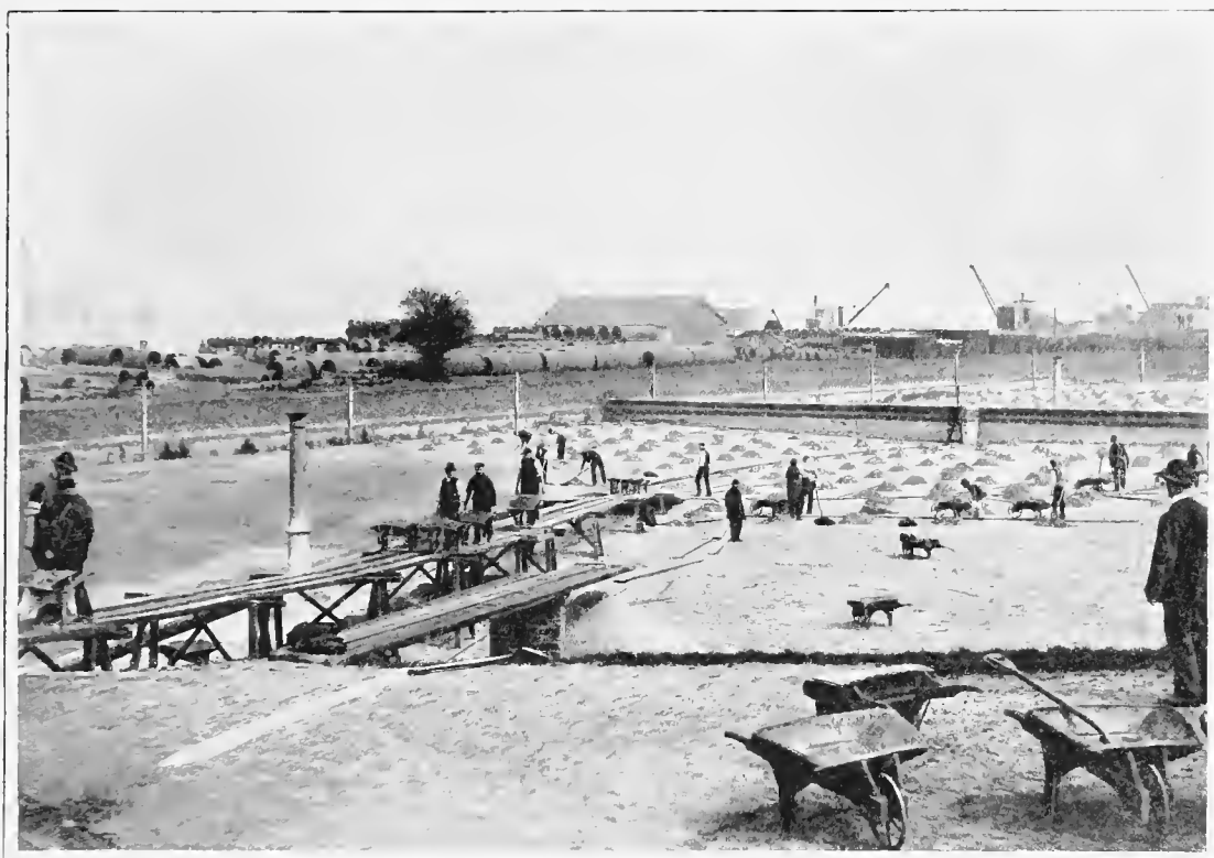
CLEANING OUT FILTER-BEDS, PATTERSEA (LAMBETH WATERWORKS)
