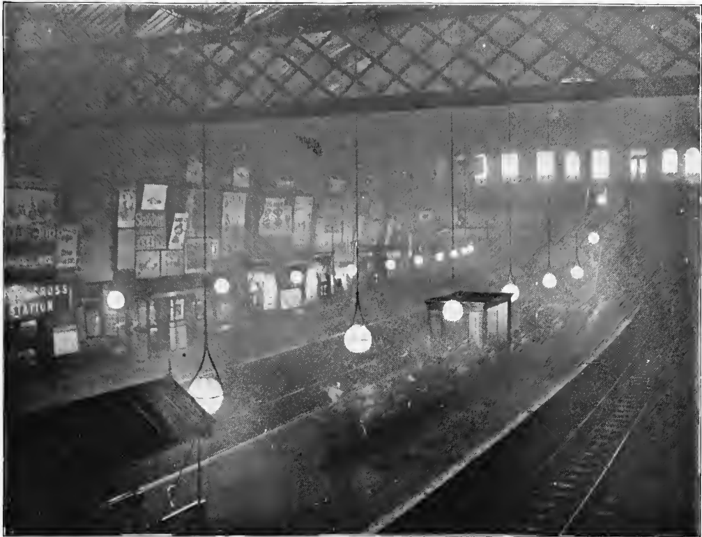
ELECTRIC LIGHTING. KING'S CROSS STATION
