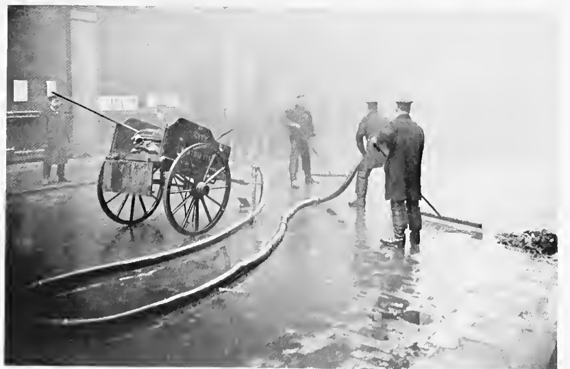
CLEANING THE STREETS WITH A HOSE
