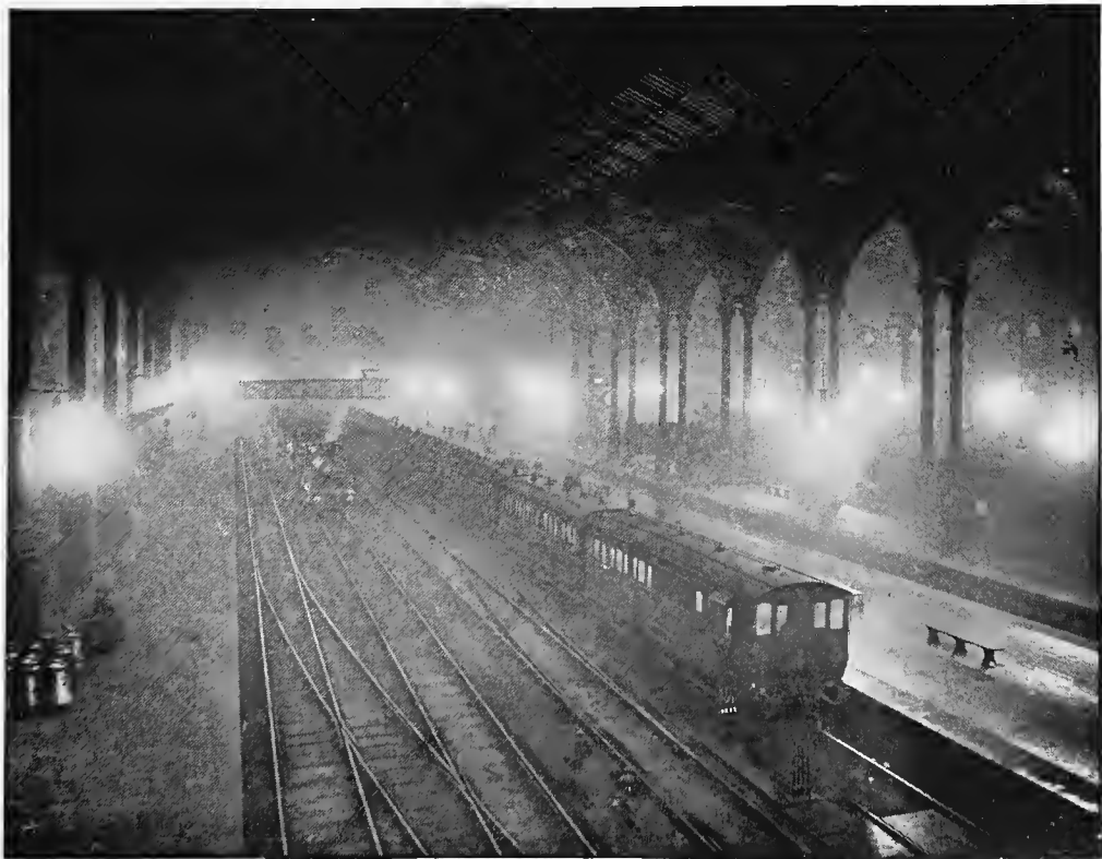
ELECTRIC LIGHTING. LIVERPOOL STREET STATION
