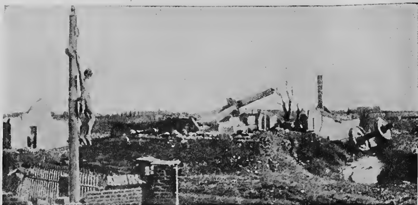
53. FARMHOUSES AND COTTAGES AND WINDMILLS DEMOLISHED. ( Page 225 )
