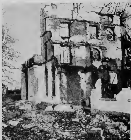
47. CHÂTEAU NEAR MALINES PLUNDERED AND BURNED BY THE GERMANS.
