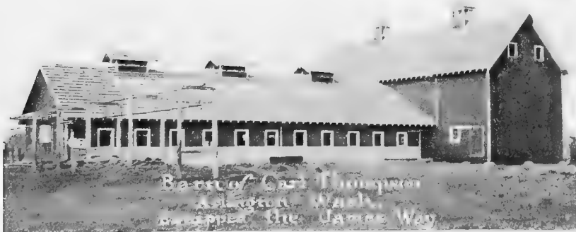
Equipped the James Way
