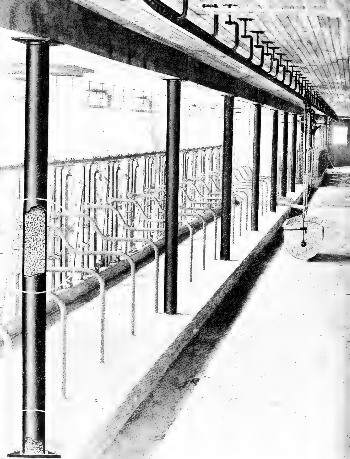
Detail of James Steel Column Red-Granite Filled
