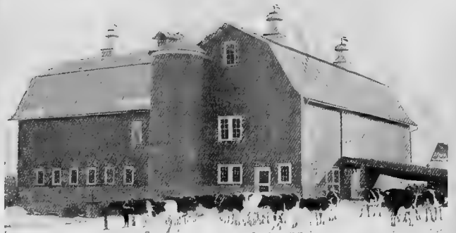
Barn of D.V. Whiteleather Columbia City Ind. Designed and Equipped the James Way
