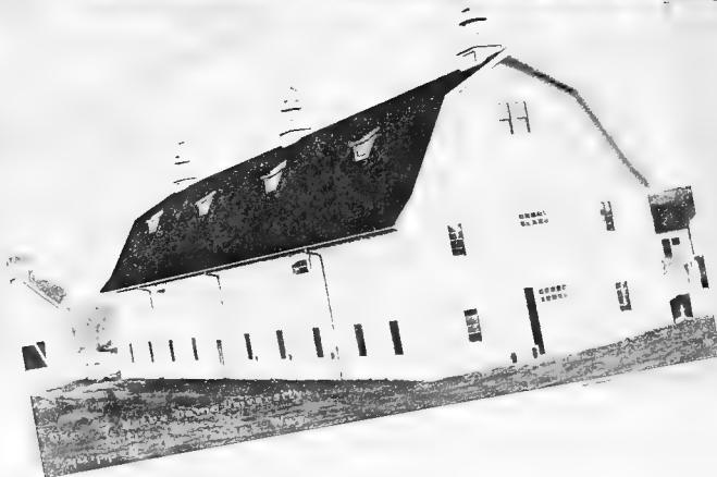
Barn of H. E. Chase - Framingham, Mass. Equipped the James Way.
