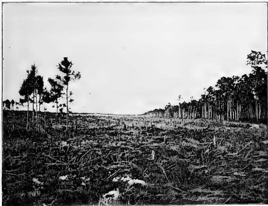
FIG. 9. — Clearing the "Pine-yard" for Sisal near Nassau, N. P.
