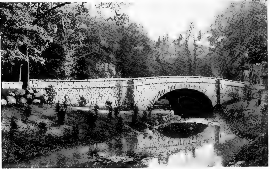
THE BRONX RIVER PARKWAY AT SCARSDALE
